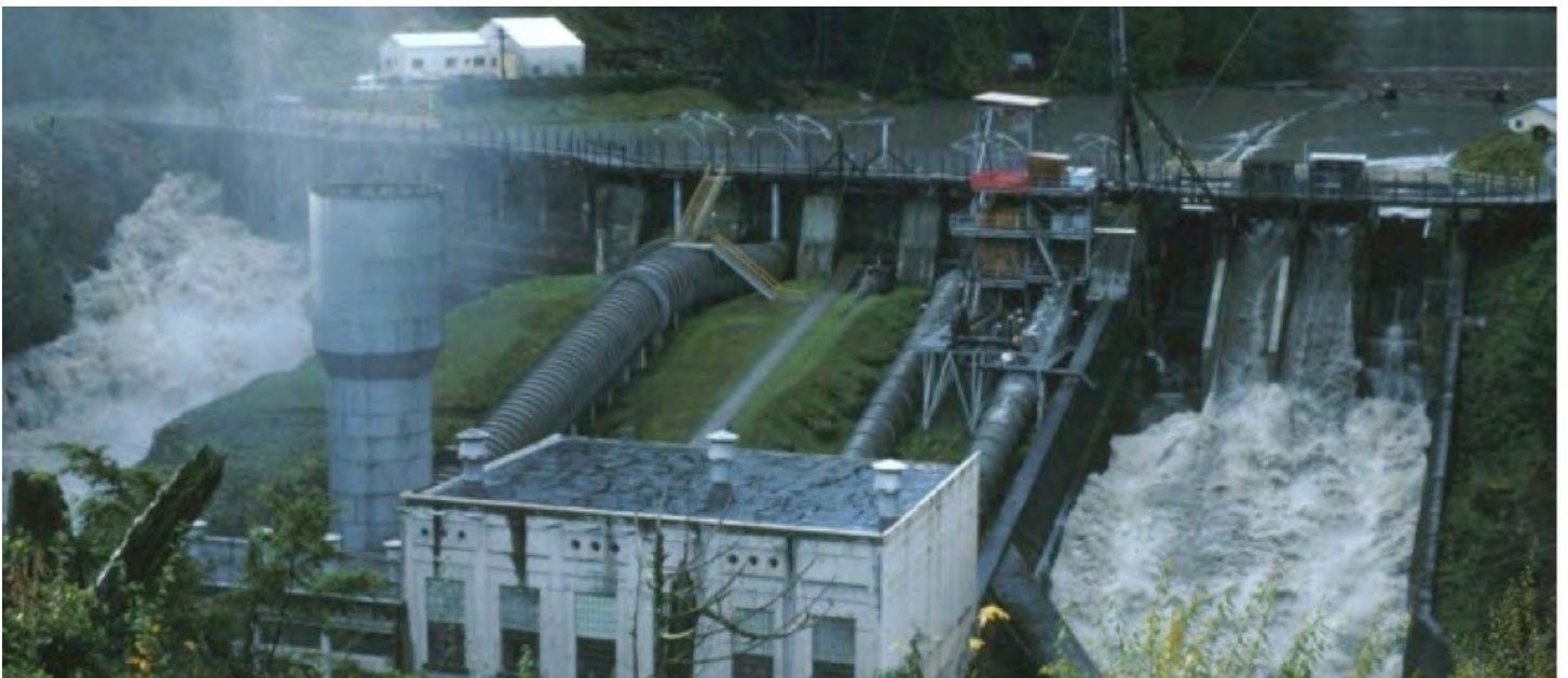
Elwha Dam before removal
