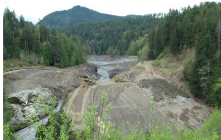
Elwha Dam Removal, 2012
