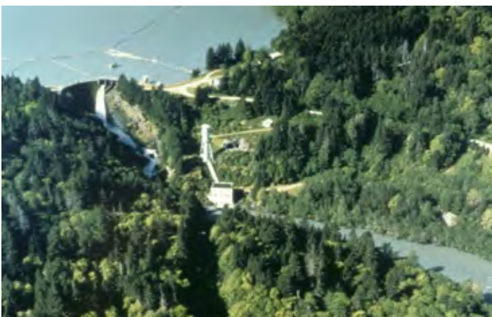
Glines Canyon Dam before removal
