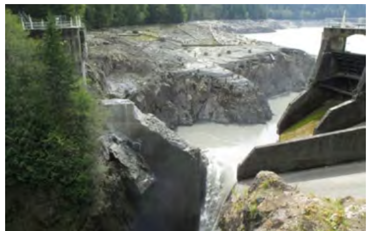
Glines Canyon Dam, 2012
