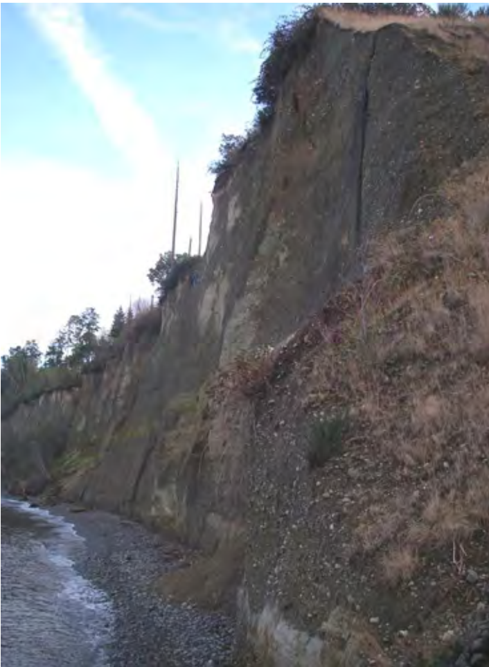
Current site conditions east end cell 304
