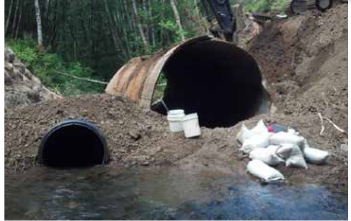
Upstream diversion pipes direct water around the worksite. Photo: Nicole Rasmussen
