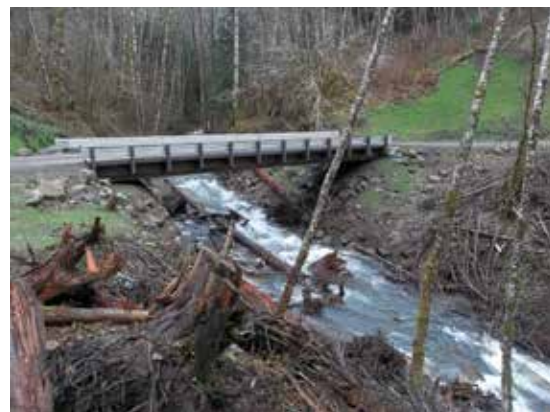
After: The new bridge opens up more than three miles of stream habitat year-round to salmon. Photo: Carl Chastain
