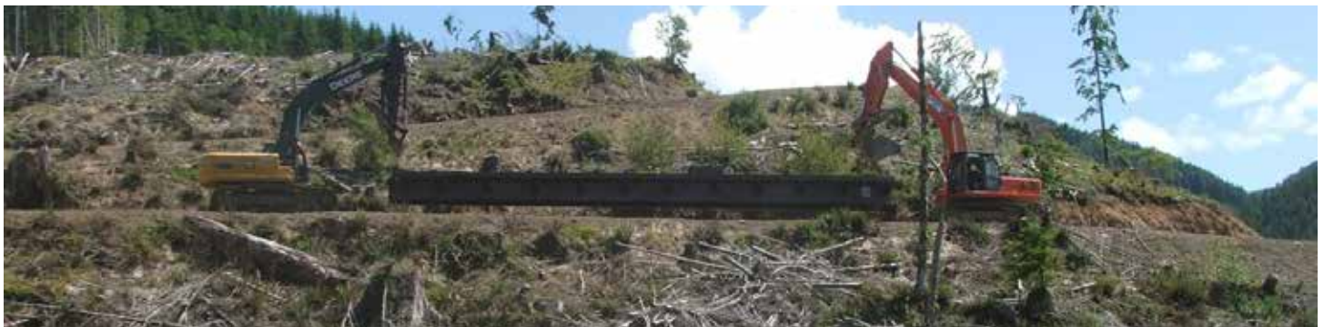
The 70 x 17 foot bridge was wider than the road in some locations and required skilled and coordinated maneuvers to deliver and place it over Camp Creek. Photo: Carl Chastain
