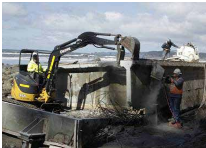
Workers section the concrete casing into smaller pieces on March 18, 2013. Photo: NPS/ John Gussman.
