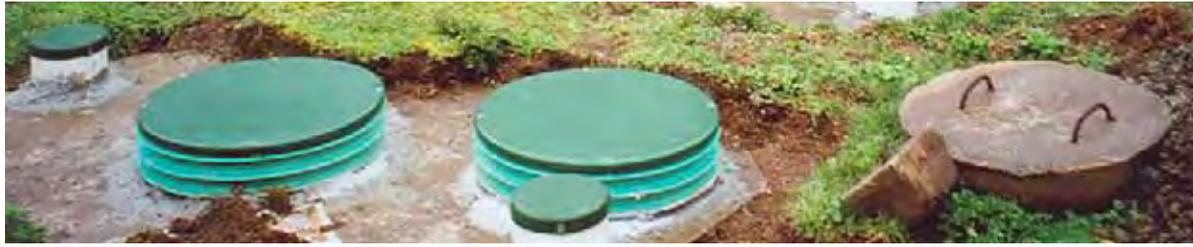
The above photo shows a proper installation for this style of septic tank – two manhole access risers and two smaller risers to access the inlet and outlet baffles of the tank. This is a very shallow septic tank installation, you will need to dispose of the concrete covers.
