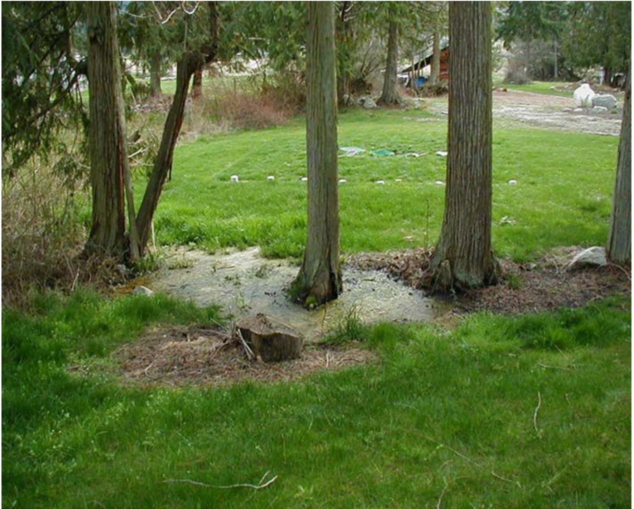
Image: Failing drainfield
